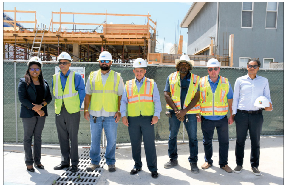
► Minister Hew with Public Works Department and Cayman Structural Group in front of Apprentice Training Facility construction site
