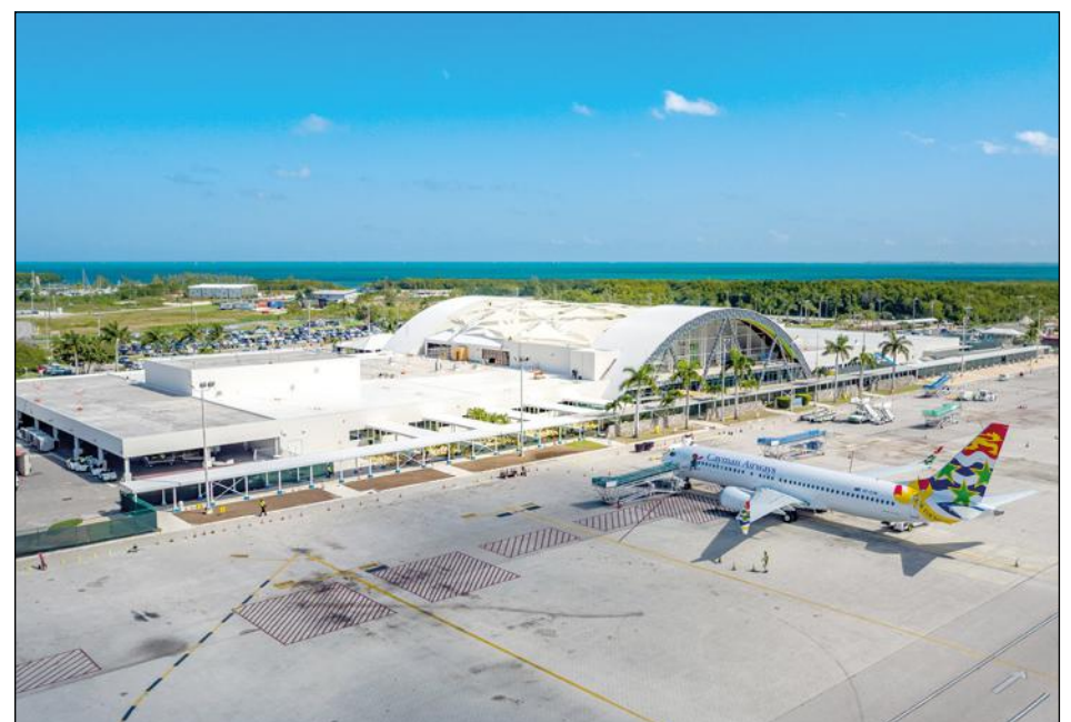
► Airside views of the new Owen Roberts International Airport
