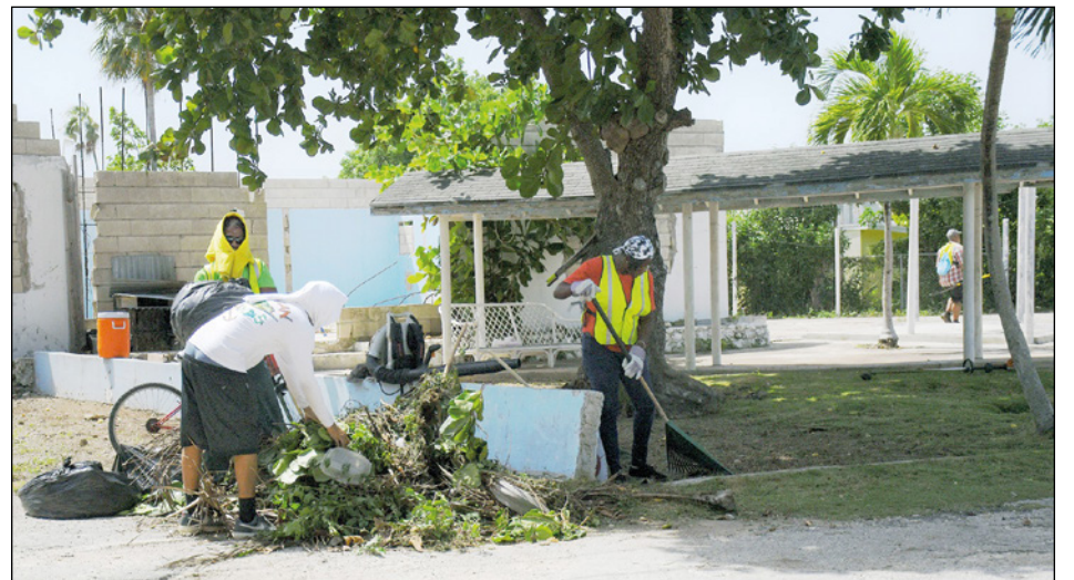
► Government property in West Bay gets spruced up and cleared by NiCE workers with rakes and leaf blowers
