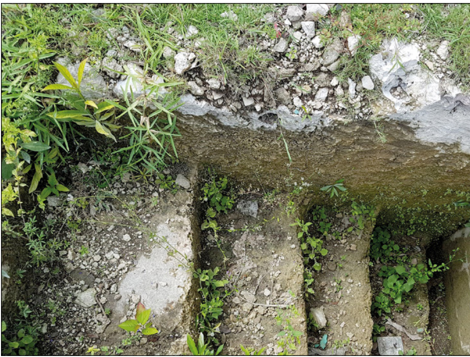
► Detail of the wattle and daub with limestone wall and ironwood posts
