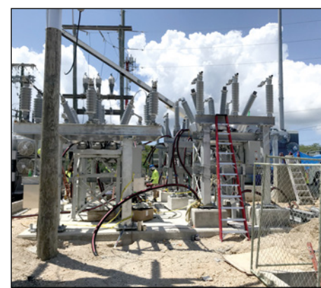
► Work being carried out to upgrade the Bodden Town substation
