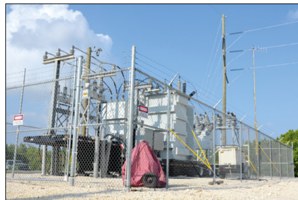
► In June 2019, construction will begin to replace the existing Prospect Substation
