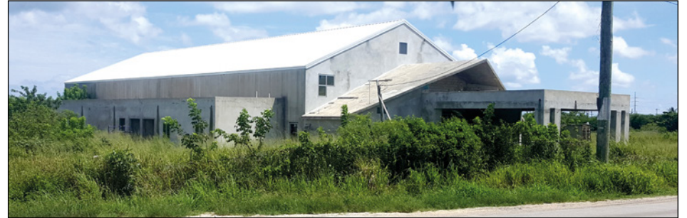
► Bodden Town Hurricane Shelter In Progress
