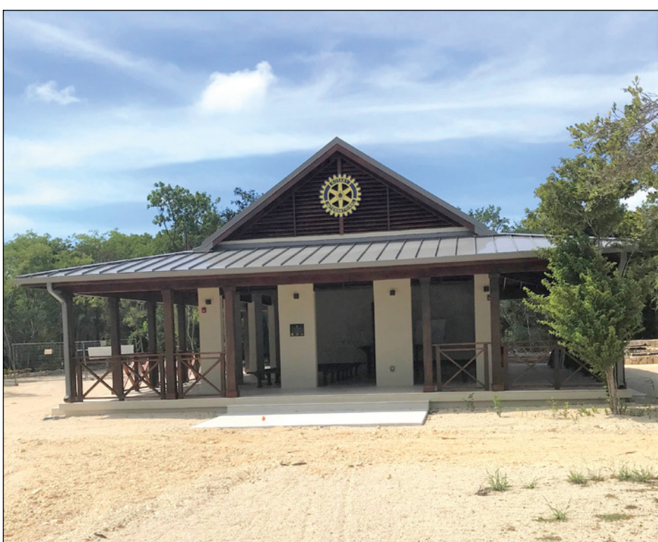
► Exterior of the new Rotary Schoolhouse in the Children's Garden classroom at the Queen Elizabeth II Botanic Park
