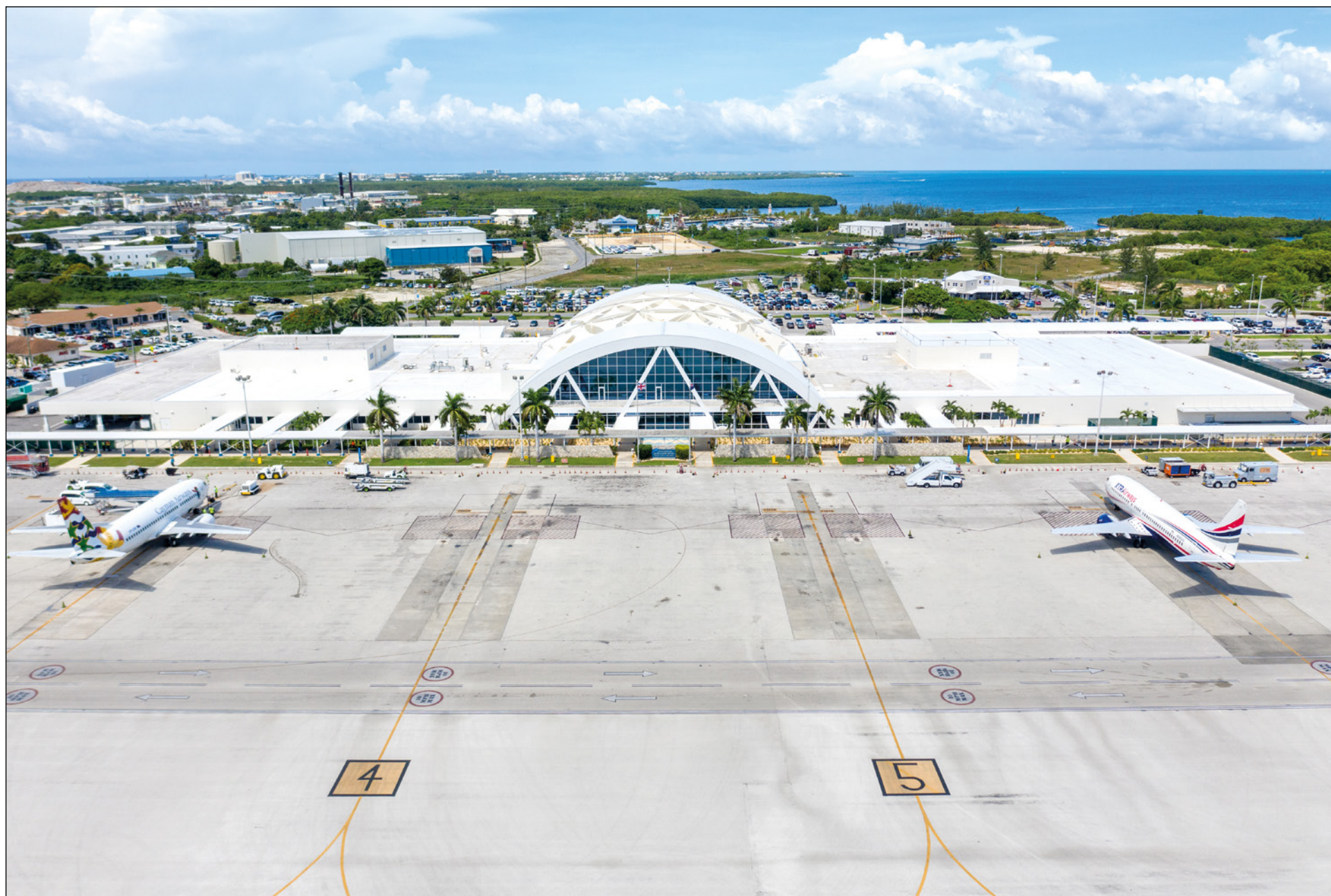
► Works on rehabilitating the runway at Owen Roberts International Airport began in early February 2020 and will take approximately five months to complete
