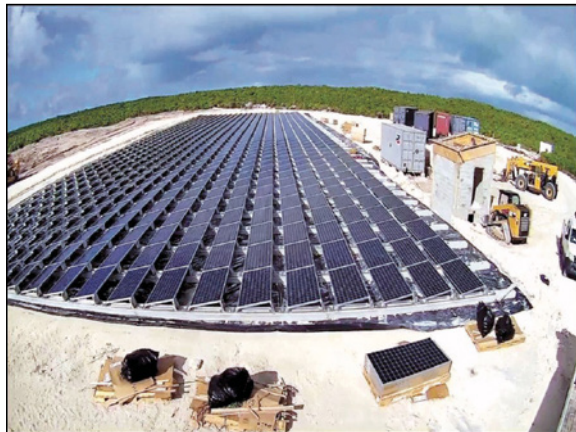
► The Bahamas is laying solar panels in Abaco
