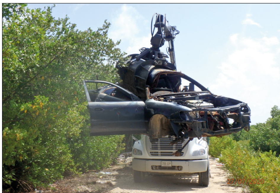
► Removal of Derelict Vehicle
