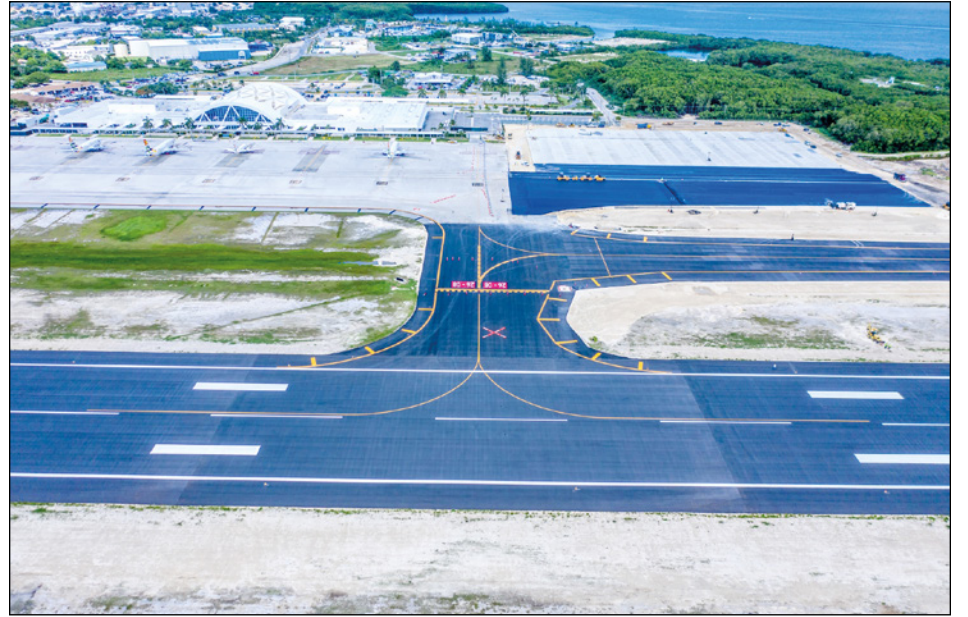
► New junction of Taxiway Foxtrot and Taxiway Gulf
