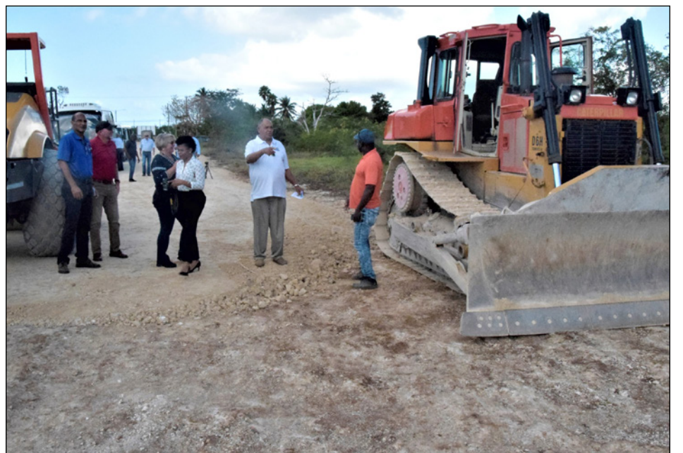
► New extension to Rex Crighton Boulevard, looking east
