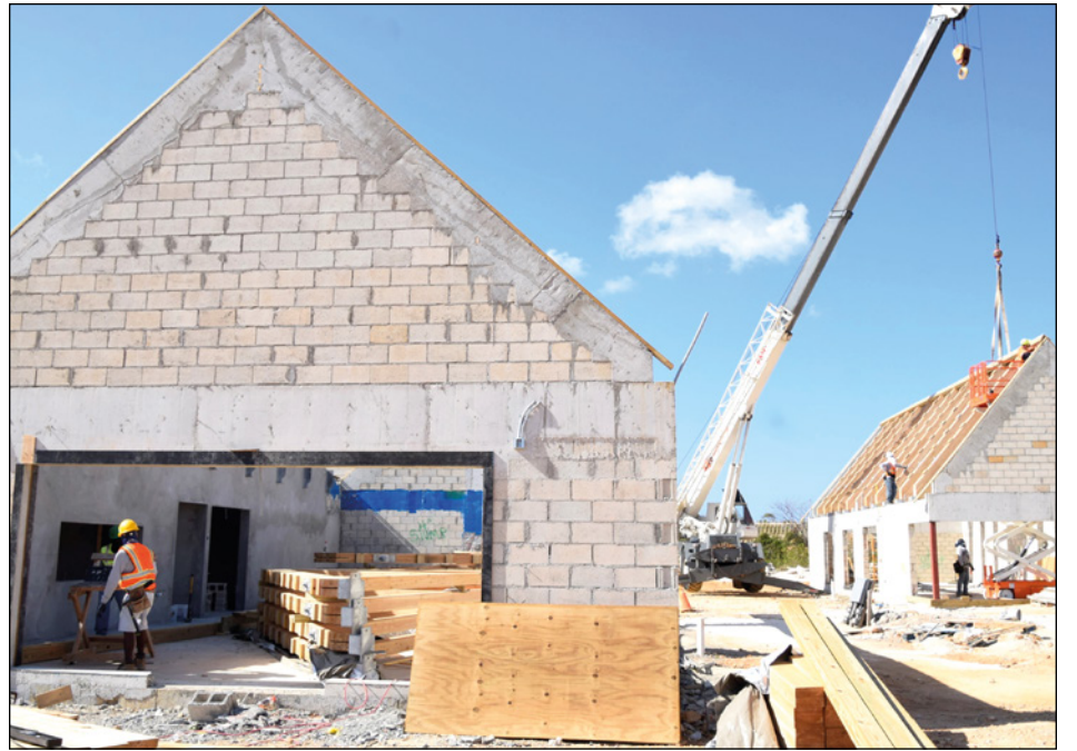
► Construction of the new facility
