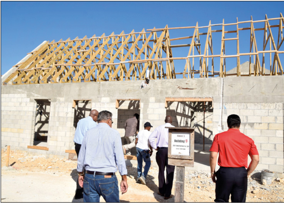
► Looking around one of the new cottages
