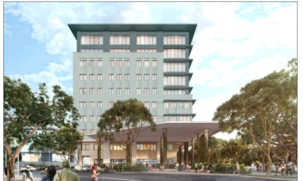
► The ceremonial raising of the beam during the "topping out" of 60 Nexus Way
