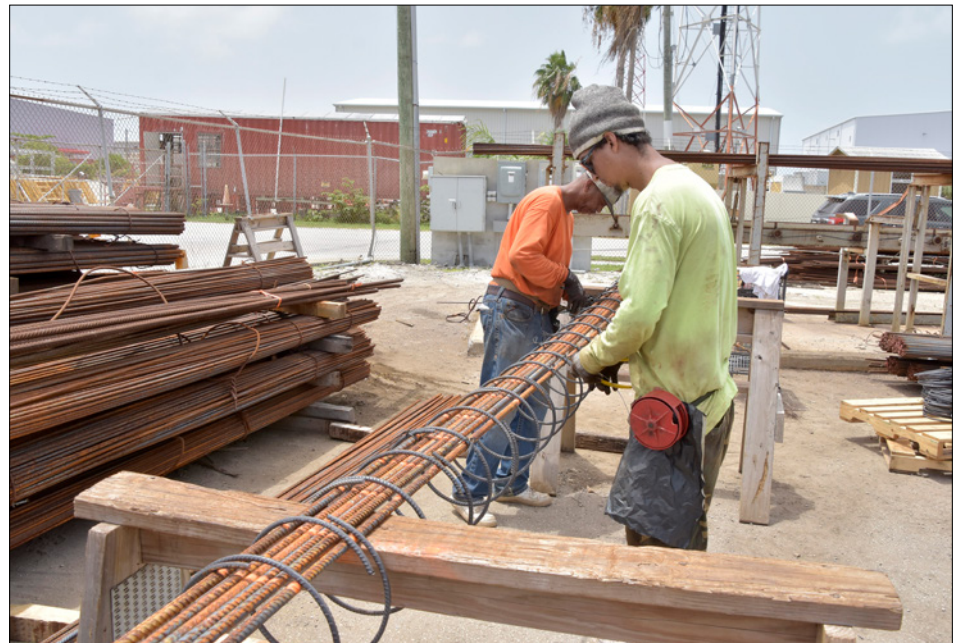
► Employees at Cox Lumber assemble the rebars, saving time onsite
