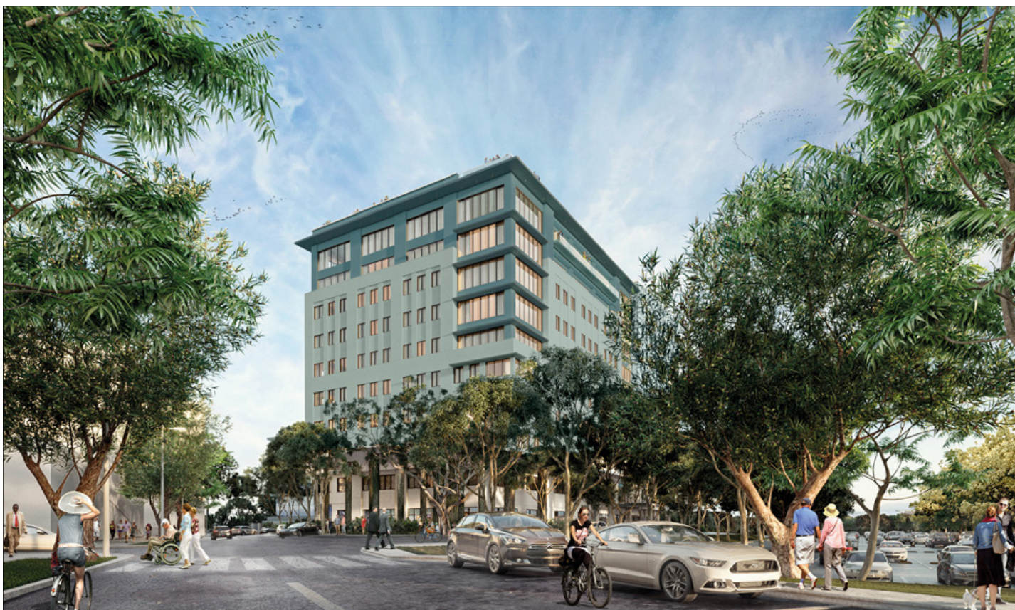
► 60 Nexus Way, which mixes urban and tropical design features with modern infrastructure, is the ideal location for commercial operations.
