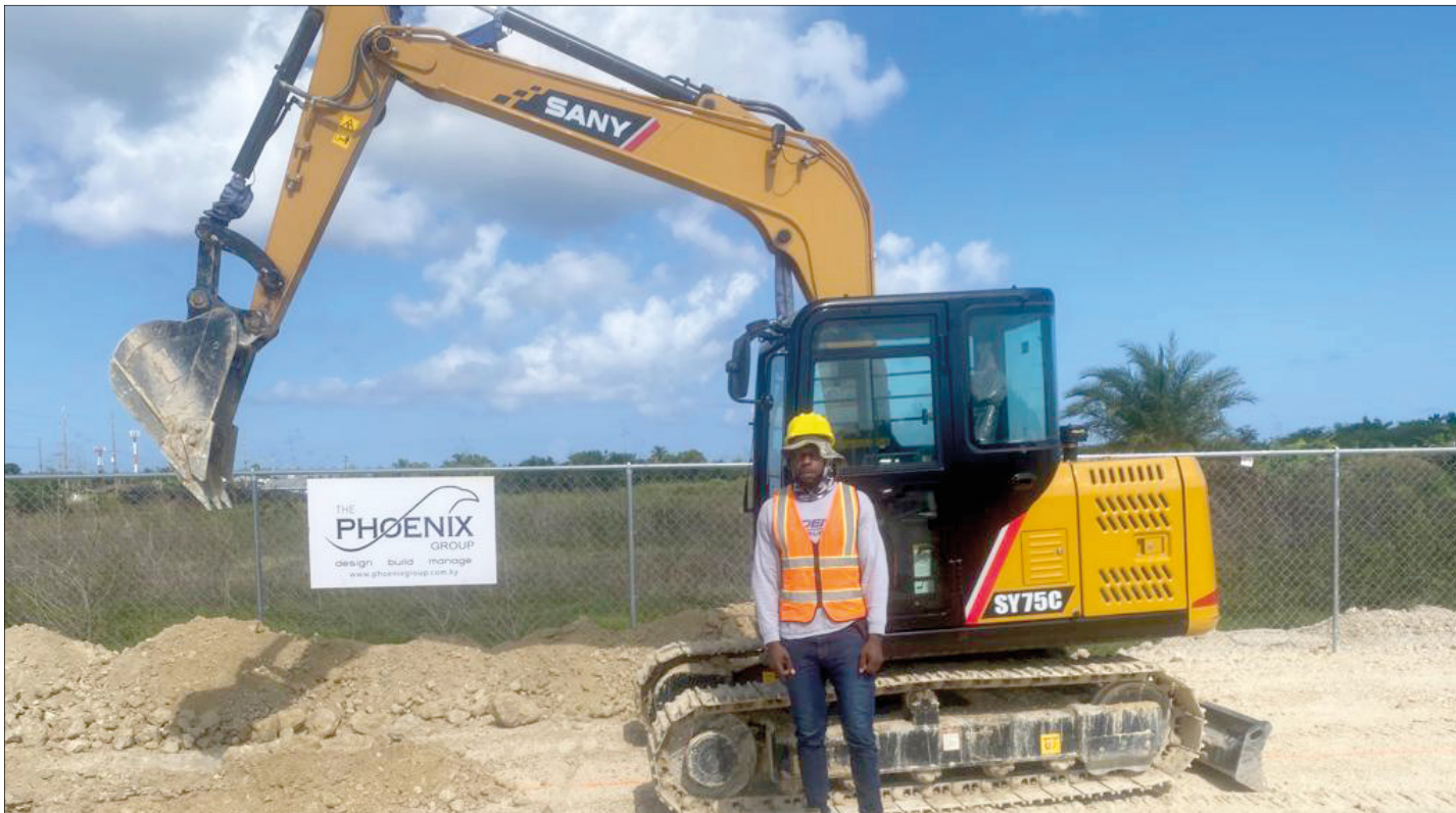
► Chris Myles on site with Phoenix Construction after receiving his Excavator Certification from the Inspire vocational training programme.
