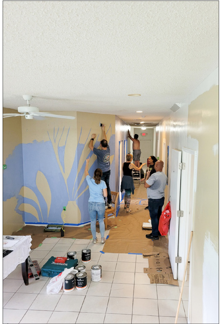
► Renovations to Phoenix House, 2023
