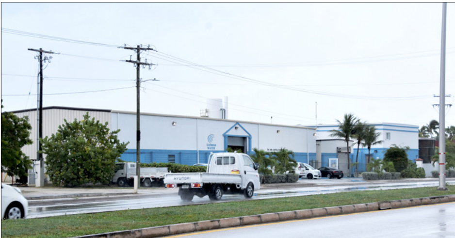
► The Abel Castillo Water Works at Governor's Harbour
