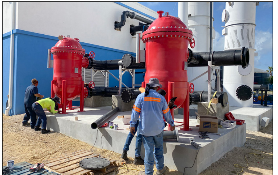
► The Cayman Water Company – plant and workers
