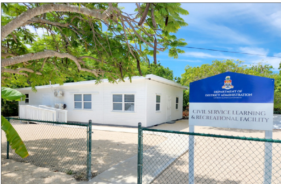
► Front exterior view of the Civil Service Learning and Recreational Facility in Cayman Brac
