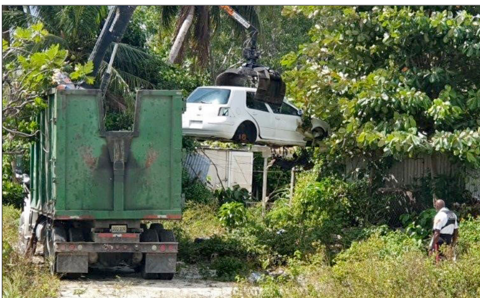
► Removal of Derelict vehicles
