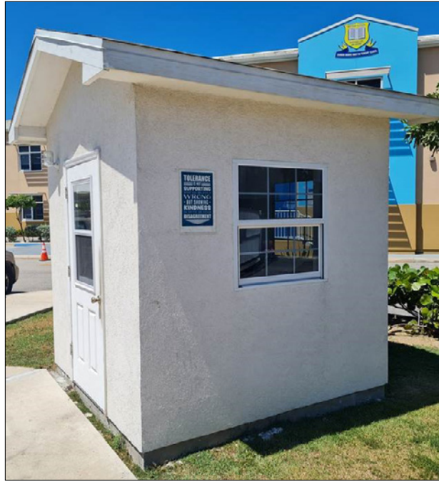
► The new security booth at Marie Martin Primary School.
