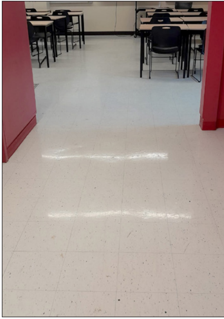
► A newly tiled section of the Clifton Hunter High School.
