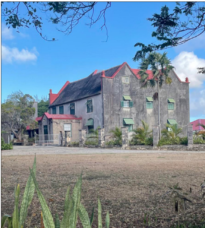
► Drax Hall has caused much controversy
