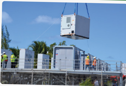
2024 – Installing batteries at our Battery Energy Storage Systems site
