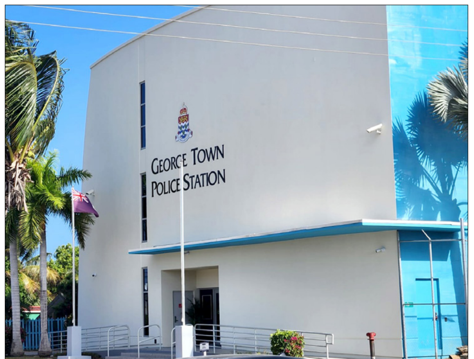
► 19 Eastern Avenue, which was formerly One Technology Square and otherwise known as the Flow Building, will be the new home for the RCIPS in George Town as of April 9th.
